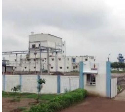
Dahej SEZ Plant
