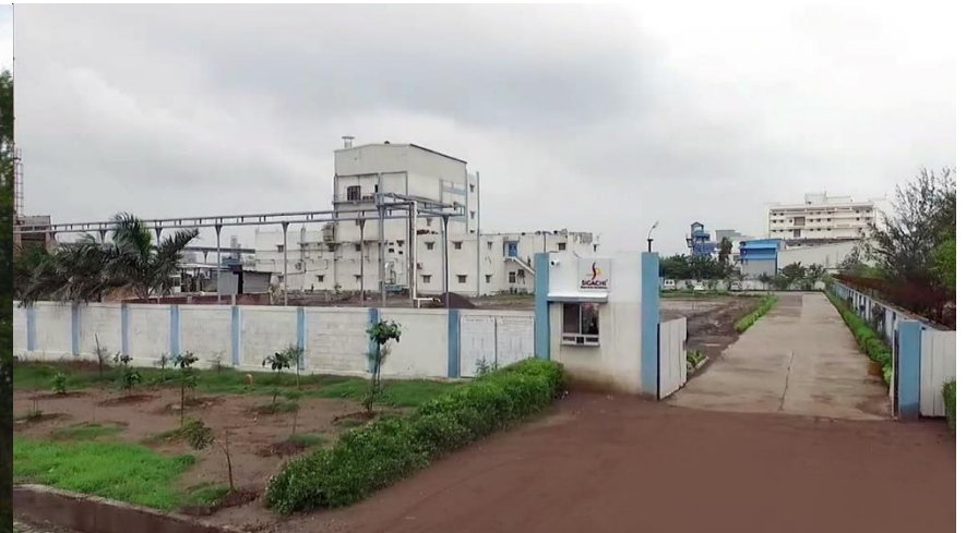
Dahej SEZ Plant
